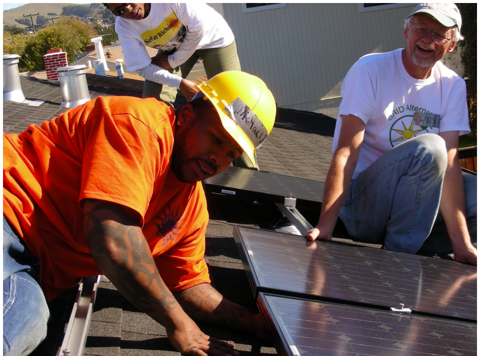
Participants with Richmond Works install a solar panel. Photo: Kirsten Schwind.
